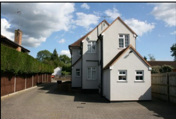
Rear of main building
