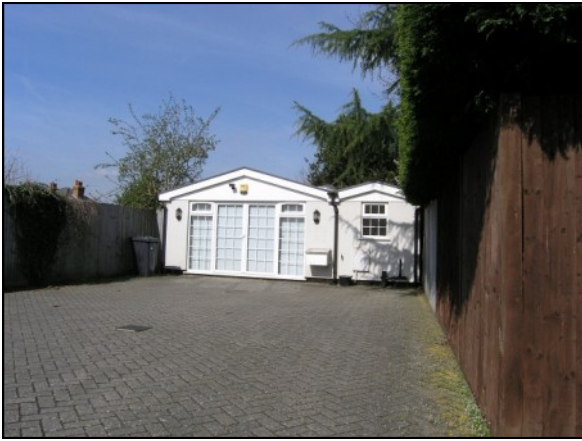
Annexe office building
